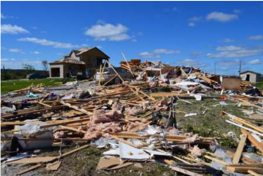
Credit: David Sills, Northern Tornadoes Project (EF3 tornado damage near Ottawa CA, 21 Sep 2018)
